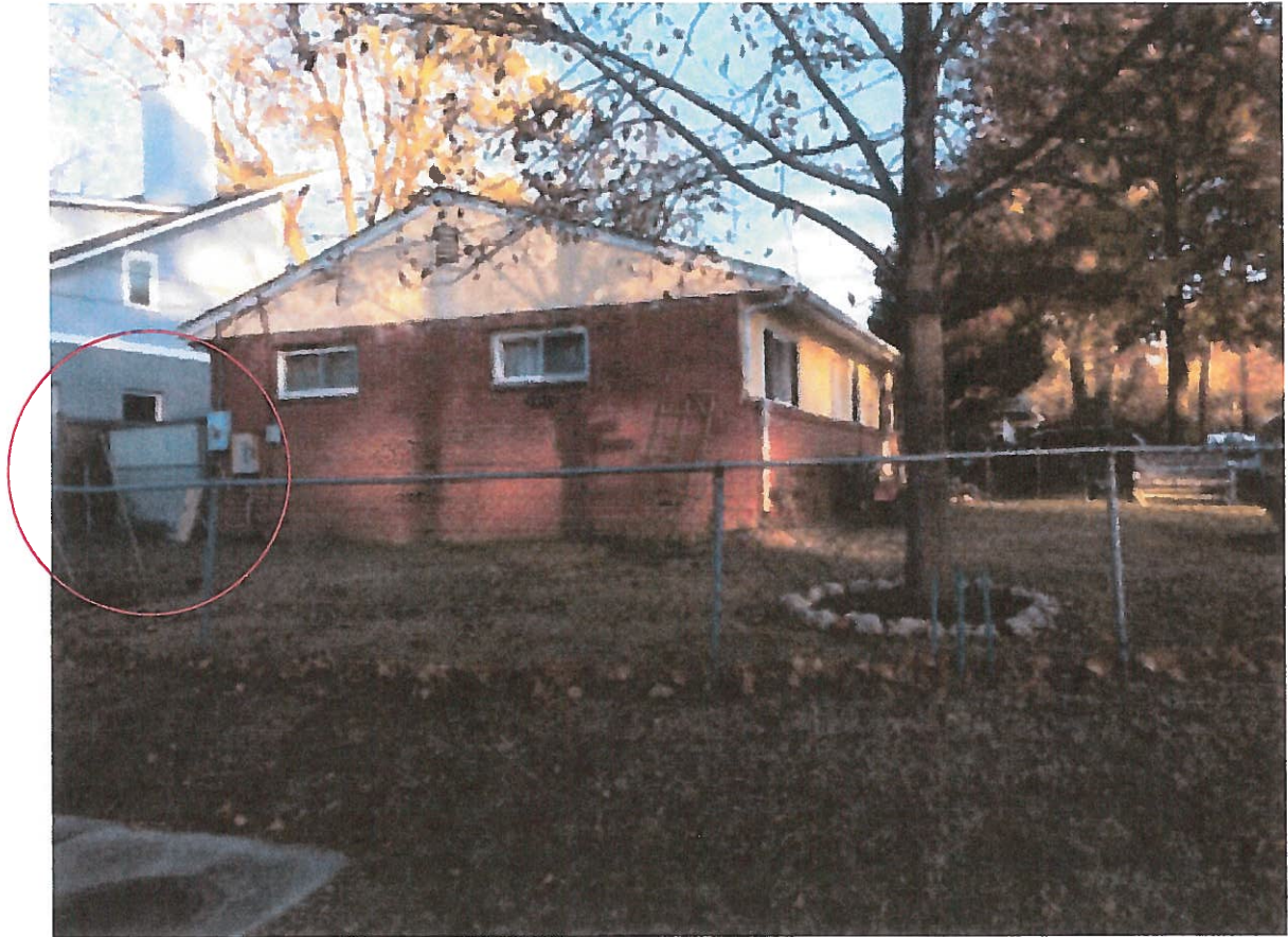
Views of shed from street
