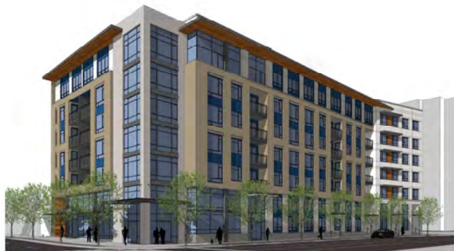
View of proposed development from North Glebe Road and North Carlin Springs Road
