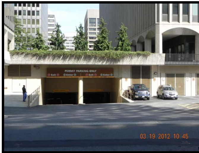
Garage entry from 20 th Street South with Center Park above
