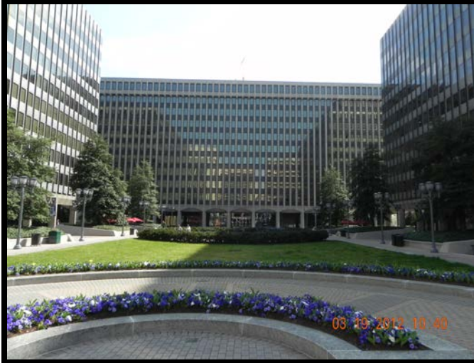
Mall II, III and IV buildings from Center Park
