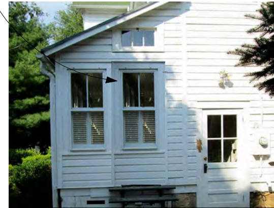
New Window to be wood, painted True Divided Light Mullions, Trim & Sash to match (Photo Enhanced to show proposed)
