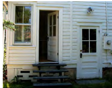
SIDE STEPS (To Be Removed )
