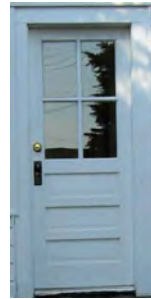
New North Side Door Wood Custom Painted as Existing
