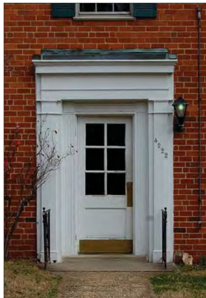
Right: examples of appropriate entrances and doors
