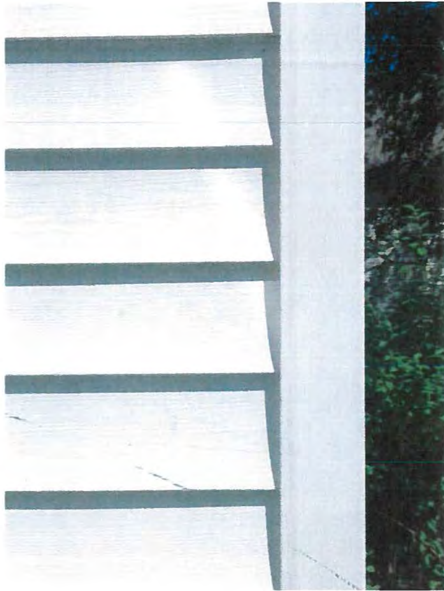
Close -Up View of Current Vinyl Siding
