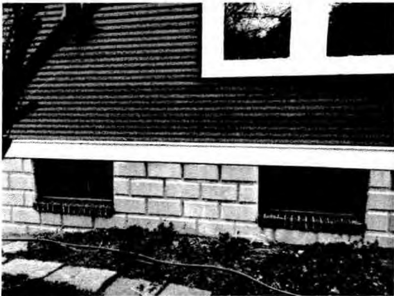
(Window replacement on right)
