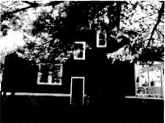
North Side of House, Existing – Proposed Egress window on far left side of photo
