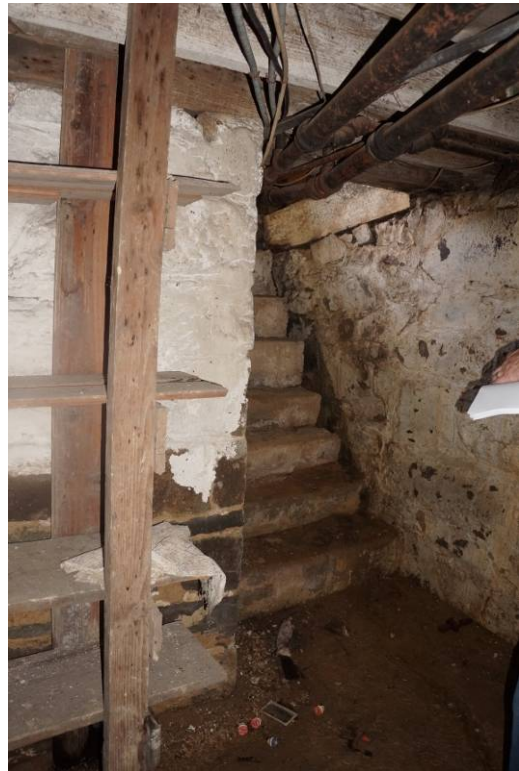
Figure 7. Existing basement stair.
