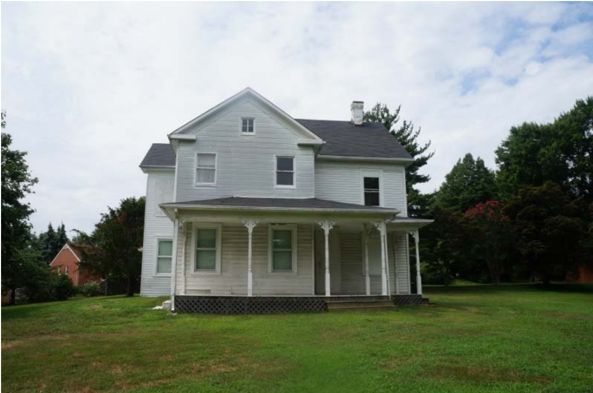
Figure 2. The front of Reevesland farmhouse, looking west.
