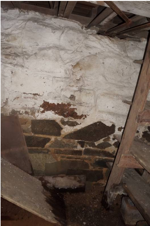
Figure 6. Existing basement stone wall.
